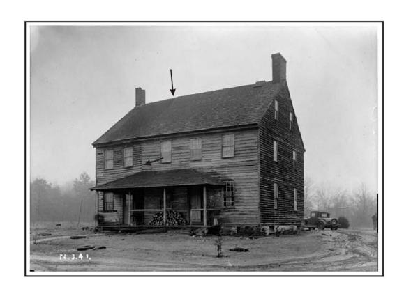
**Figure 3.4:** 1938 HABS, Photograph of the Tavern at Cedar Bridge (Survey No. N.J. 41). View Southeast. Arrows denote structural addition line.
